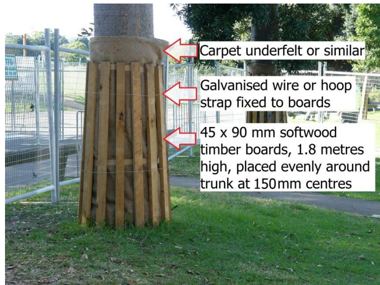
Figure 3 – Detail of Trunk Protection
